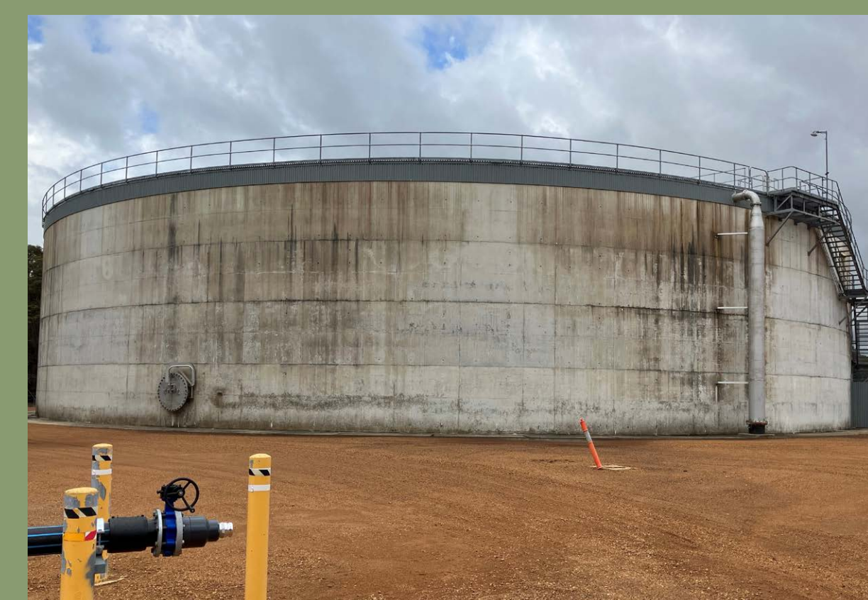
Decommissioned Water Corporation water storage tank, Margaret River (Credit: Lorraine Duffy)
